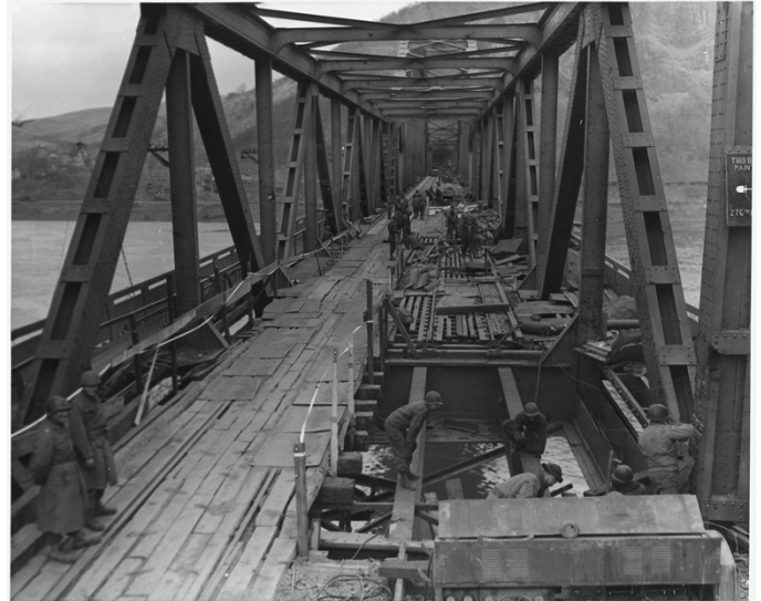
Combat engineers at work on the bridge on March 17, 1945, just hours before its collapse. US Army photo.
